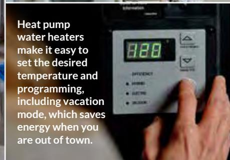
Heat pump water heaters make it easy to set the desired temperature and programming, including vacation mode, which saves energy when you are out of town.
