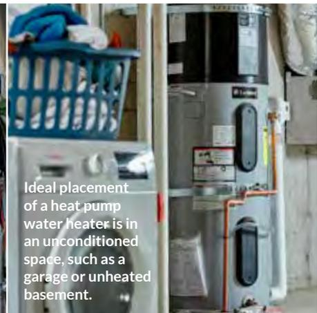
Ideal placement of a heat pump water heater is in an unconditioned space, such as a garage or unheated basement.
