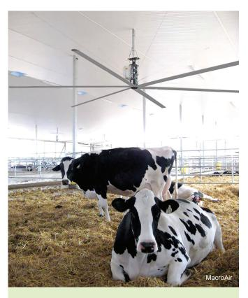
A 24-foot HVLS fan will move as much air as six standard industrial high-speed fans and consume only one-sixth the energy. In a typical dairy-free stall barn, HVLS fans are placed over the feed alley every 35-60 feet, depending on the fan size.
